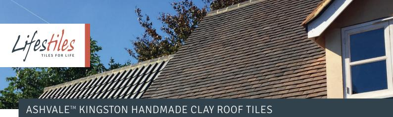
The Ashvale clay roof tile is one of the few handcrafted tiles available on the market today that still involves hand forming and is not entirely manufactured on a machine. Each tile is made with varying cambers producing an individuality in appearance and with an excellent selection of colours and blends, there is in Ashvale to suit everyone's requirements.any roofing project.
